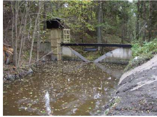
(b) Looking downstream.
