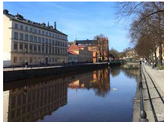
(2) Directly upstream Islandsfallet.
