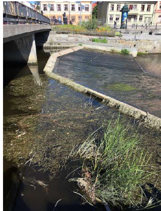
(b) Looking downstream.
